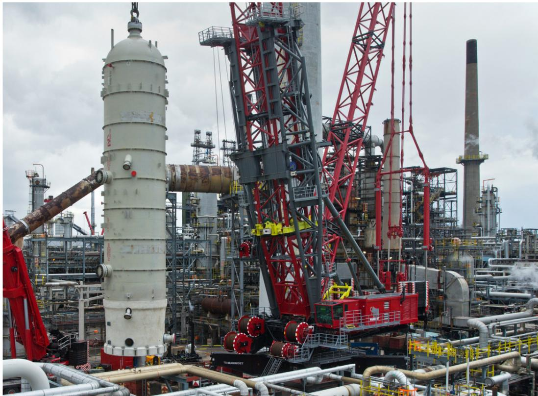
**M**ammoet recognized that a new solution was needed to better support customers for whom restricted space was limiting the scope of lifting operations. This solution would need to be assembled and operated in confined spaces but deliver the size of lifts that modular construction projects can demand. This led to the development of the FOCUS30, a vertically self-erecting crane which has been designed specifically to operate in areas with complex infrastructure and space limitations.
